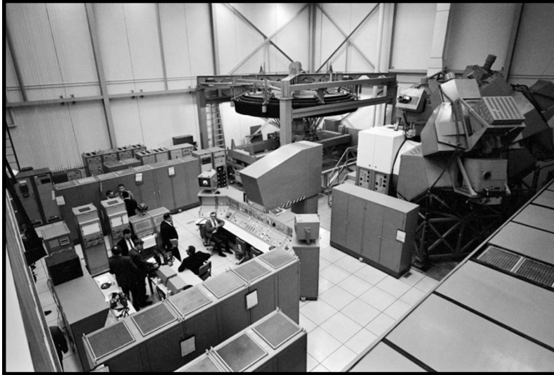
Figure 1. The landing module simulator of the Apollo program, Jackson is sitting at the control panel on the left below the middle of the picture, recognizable by his tie and cardigan (Image: NASA).
