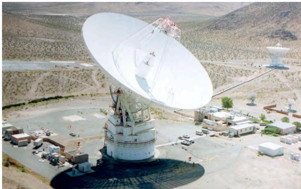
**Figure 5:** Goldstone 70-m dish (DSS-14) utilized for communication and data to/from deep space robotic missions as well as radar imagery of NEOs. DSS-14 is fully steerable to 80% of the sky (NASA, JPL).
