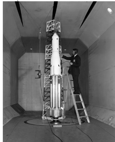
Above: Apollo Block II Saturn I aerodynamic integrity. Langley wind tunnel. Image credit: Great Images in NASA (GRIN).
